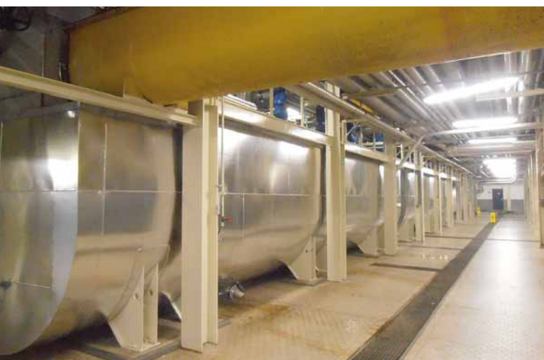
New sugar melting plant at the Dinteloord sugar factory
