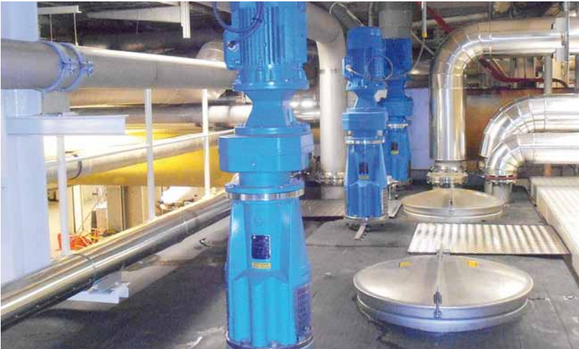
Stirrers for the first chambers
