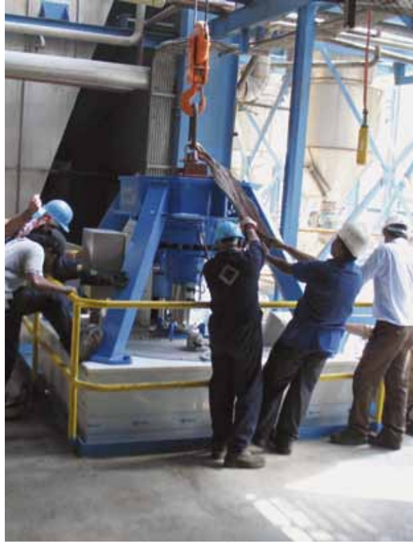
Installation of the new centrifugals
