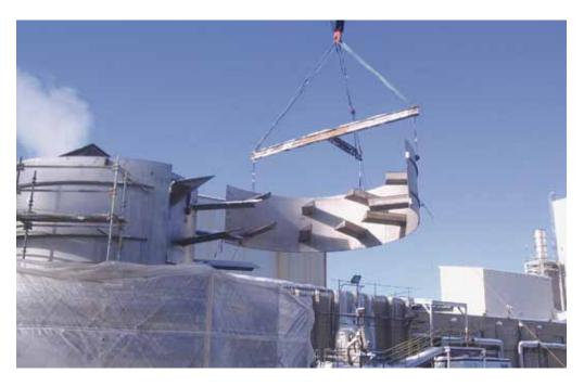
At present, BMA is building a new extraction plant on the basis of the proven "Tower 2000" extraction concept. This plant for the Moorhead sugar factory of American Crystal Sugar in Minnesota, in the Midwest of the USA, will comprise an extraction tower, countercurrent cossette mixer (CCC mixer), defoamer, sand separator, and a rake classifier. Commissioning is scheduled for the beginning of the 2011/2012 beet campaign.
