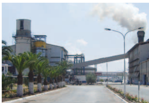
View of the main process building
