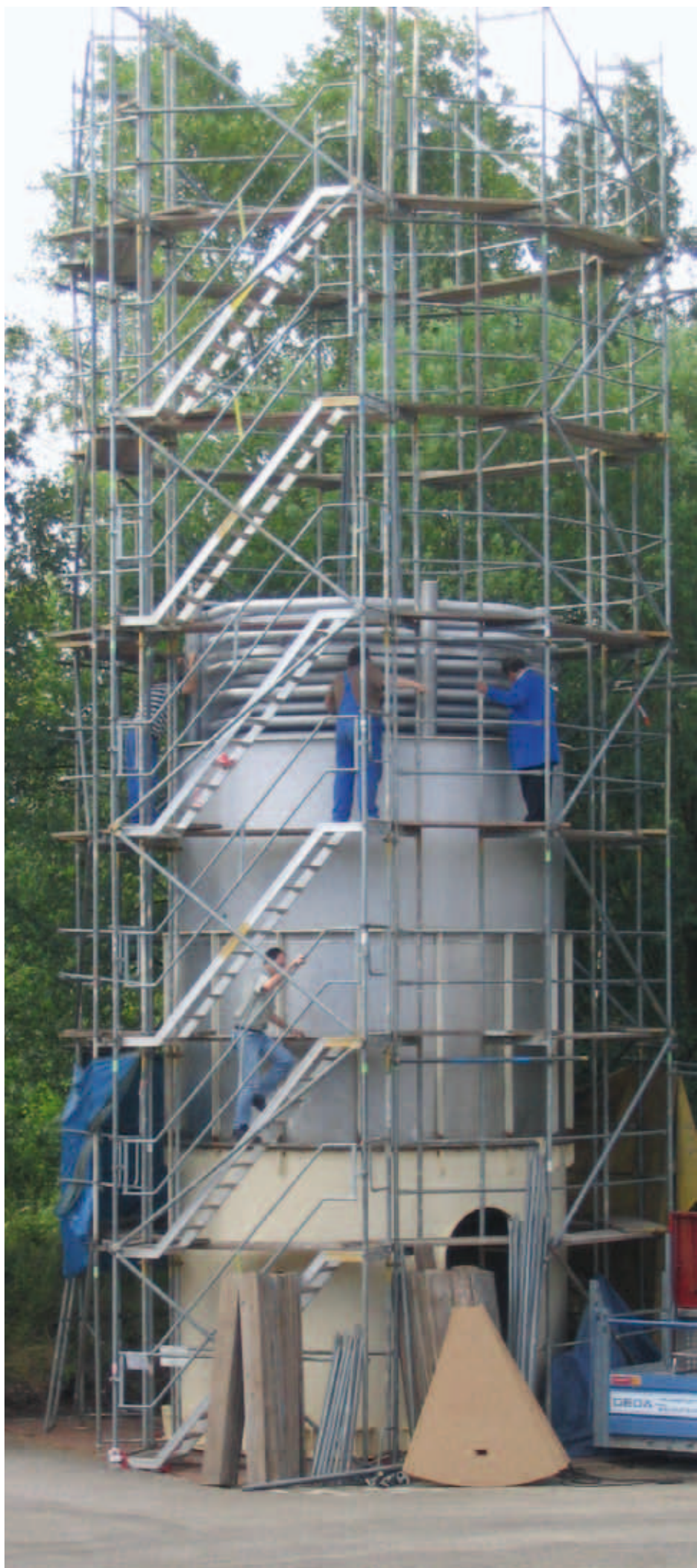
Assembly of a crystalliser
