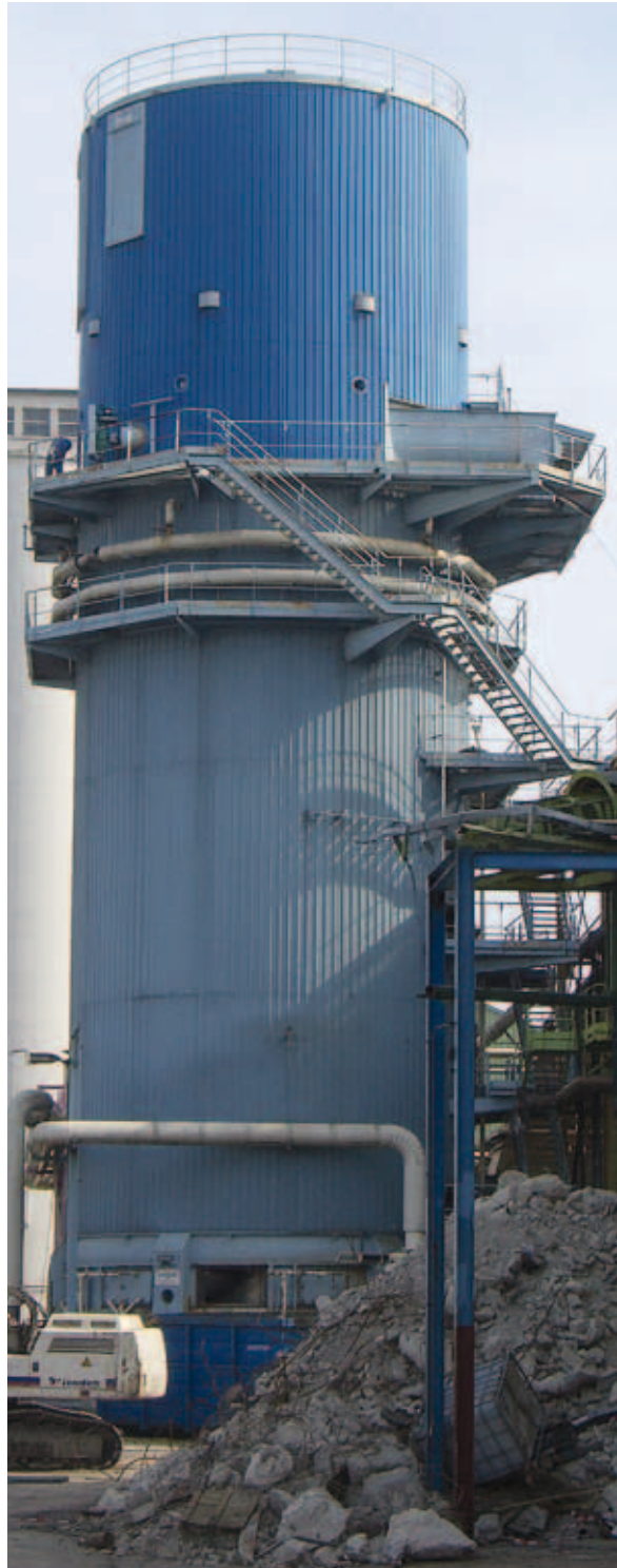
Extraction tower prior to disassembly
