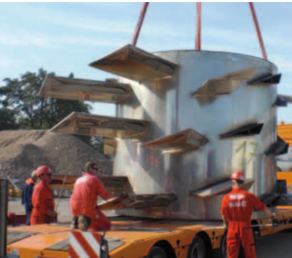
Loading of a tubular shaft
