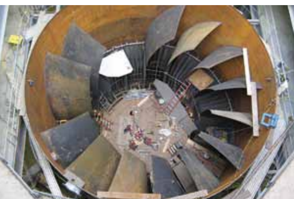
CSD-10 during construction
