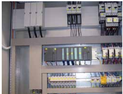
S7 control unit with Simocode for OVC
