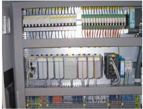
Allen Bradley control unit for rotary valves
