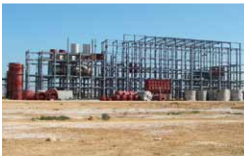
Assembly of steel structures and equipment for the main process building (as of 6 January 2009)
