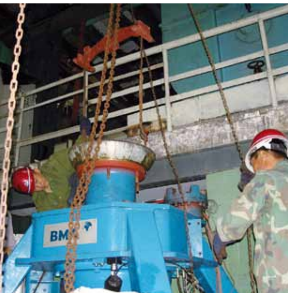
Fitters of BMA China and COFCO Tunhe during regular maintenance of a B centrifugal
